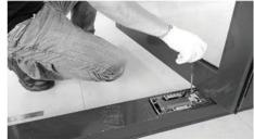
Adjust the proper closing speed of the door using the valves (6) & (5).
