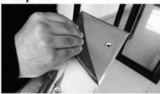
Remove the protection from the floor closer cover plate and Install it on the closer using the 4pcs screws supplied.
