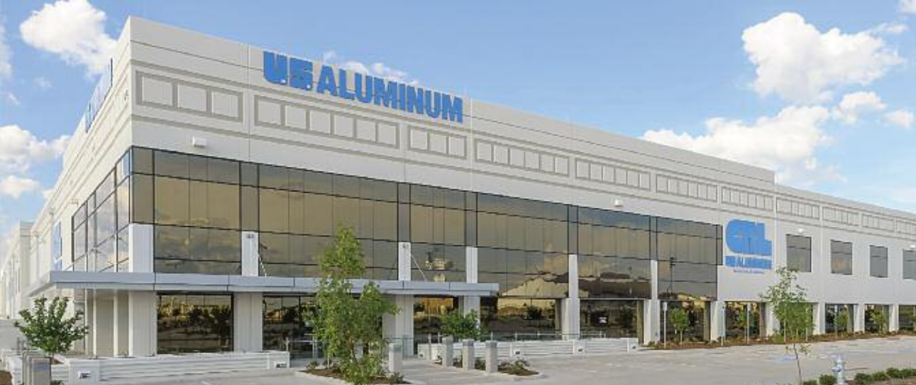
C.R. Laurence – U.S. Aluminum Manufacturing Headquarters, Waxahachie, TX
