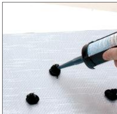
Applying mastic to mirror with Category II Tape applied to back with no holes cut out
