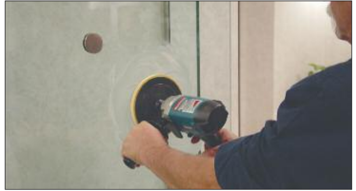
Perfect balance and properly placed handles make it possible to work with glass where it is installed, thus lowering the labor time and the cost of removing and replacing it.
