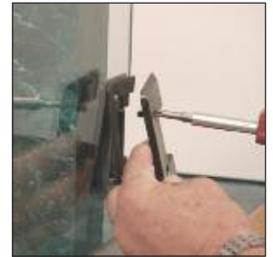
Install a new gasket and interior cover plate, replace screws, then secure in place.
