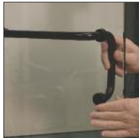
Install the new handle or knob and secure washers and set screws.
