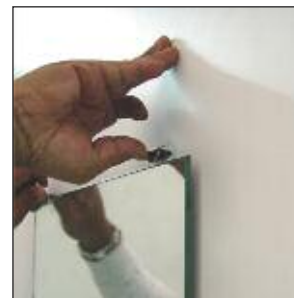
Fasten mirror into top clips
