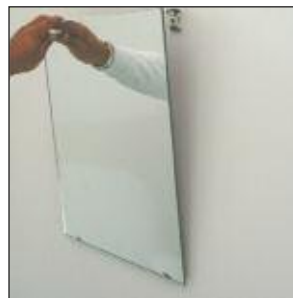
Fasten mounting brackets to wall and insert mirror onto bottom clips
