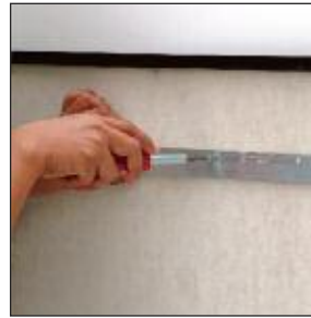
1. Attach Mounting Bracket to the back of item to be hung. For best results drill pilot holes and use screws.
