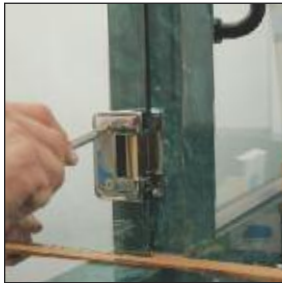
Loosen the cover plate and align the door.
