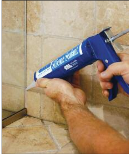
Resealing a Leaking Unit
