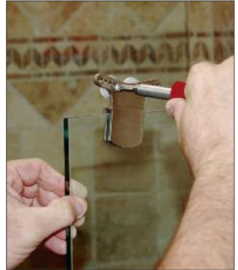
Adjusting a Sagging Door
