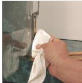
Block the door to maintain alignment and remove the cover plate. Clean glass in gasket area.
