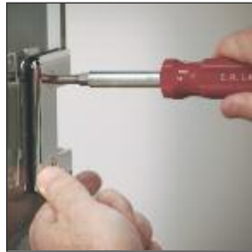
After alignment, tighten the cover plate screws by hand. Do not use a power tool, or you risk damaging the screw heads.
